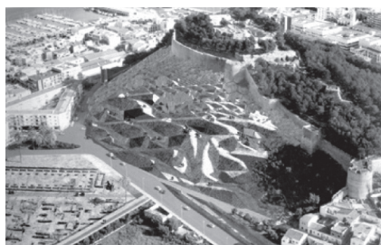
Figure 3. Vincent Gualland: Multifunctional Centre, Denia, Spain
