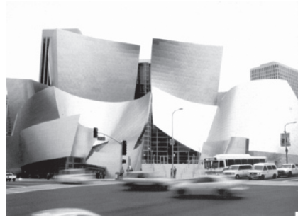
Figure 8. Frank Gehry: Walt Disney concert hall, exterior, Los Angeles
